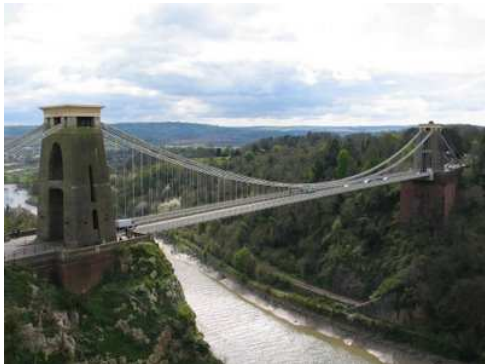
Clifton Suspension Bridge, Bristol
